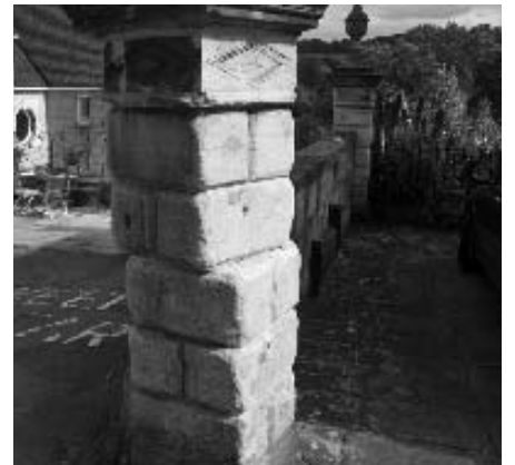
An example of damage in Vicarage Street - to a 18th century gate pillar
