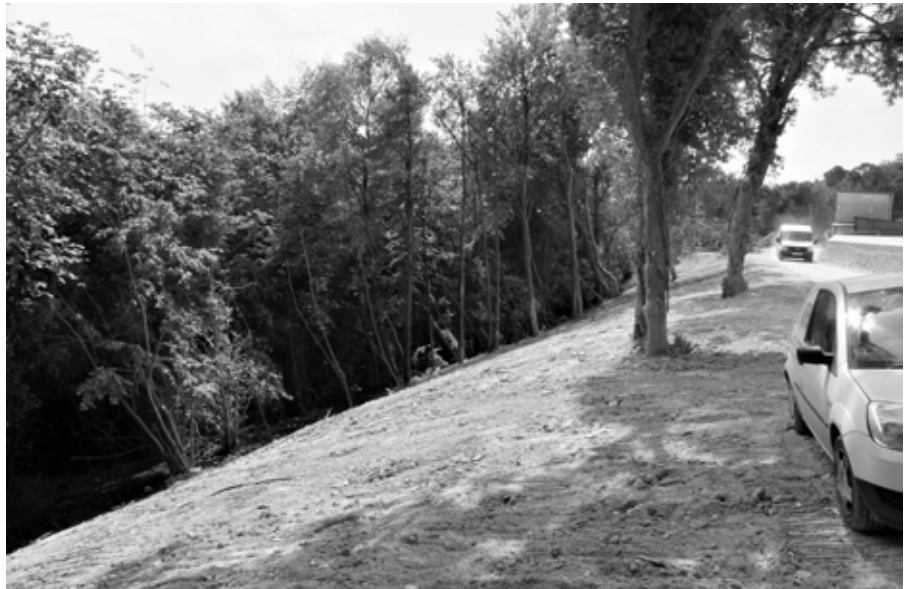
Part of the bank which used to be wooded
