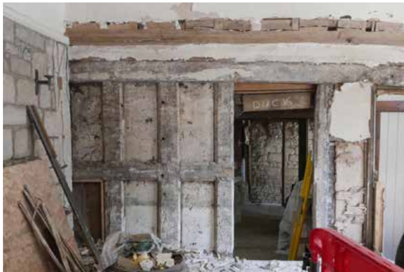
An internal view of works at Cardynham House - photo Parti Architects. The approved work aims to restore the building to its original dwelling plan.
